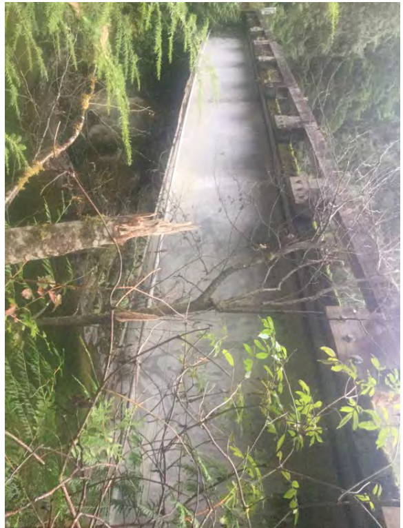
Power cable running on upstream side.
